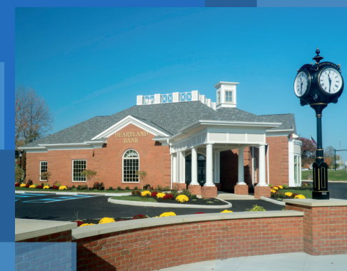
New office built to better serve the Newark community.
